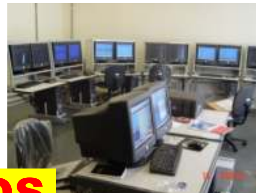
Traning center for power plants operators
